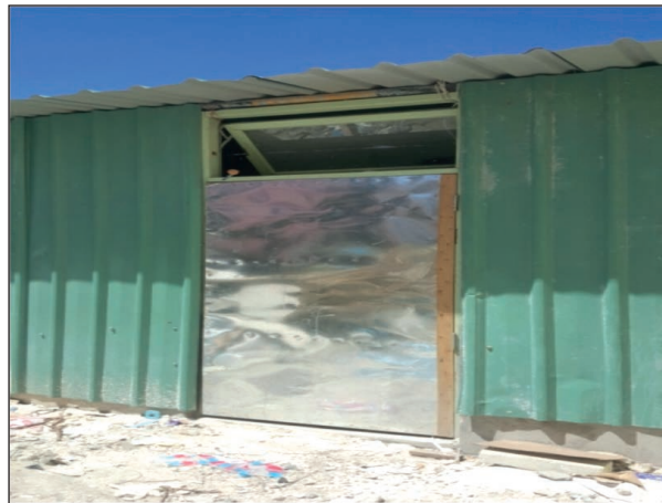
Storage area of Hulhumale Hospital
